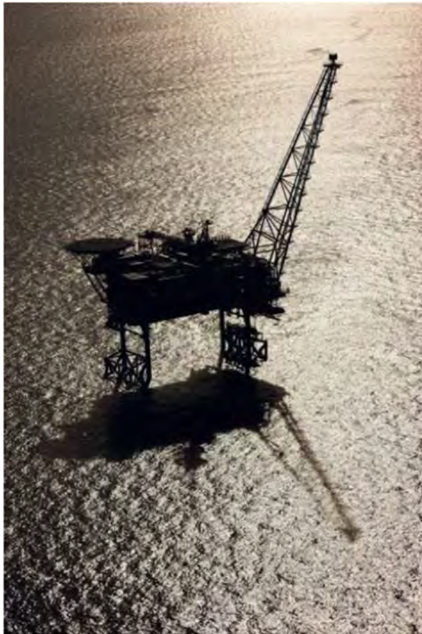
Angel gas platform North West Shelf.
