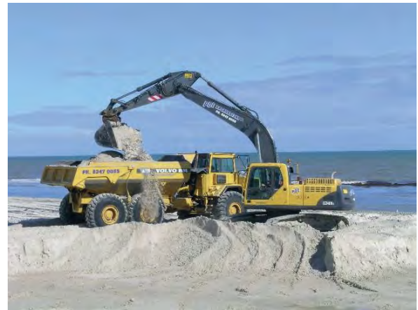
Figure 3. Sand carting by truck for beach replenishment. Photo: Coast Protection Board
