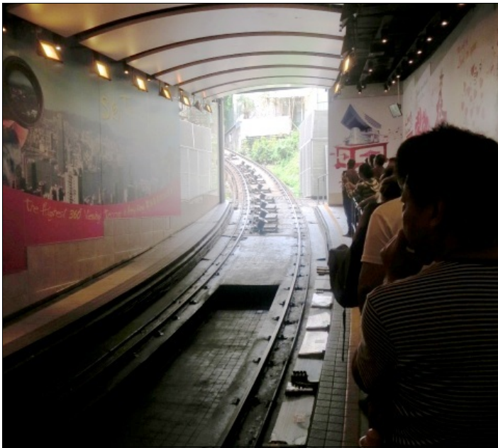
Garden Road Lower Terminus – the tramcar is out of sight around the curve. In the distance, the row of tilted rollers locate the cable when the tramcar is in the station. Photo: Brian McGrath
