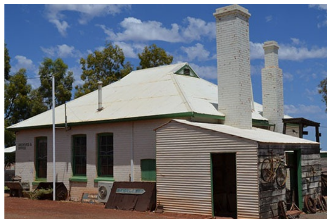
The former Assay office at the Sons of Gwalia Gold Mine – now part of the Gwalia Museum. Photo - source, Gwalia Museum
