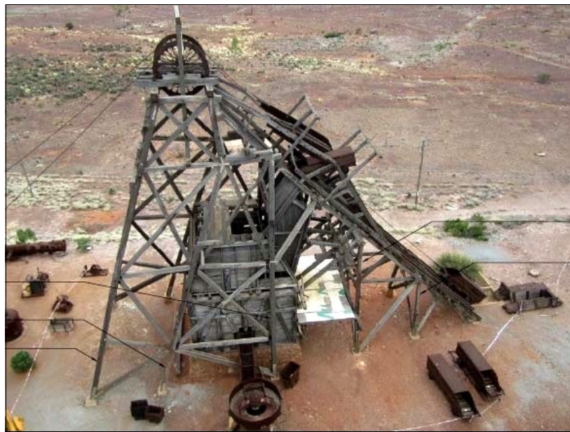
The Gwalia Headframe 2012.
