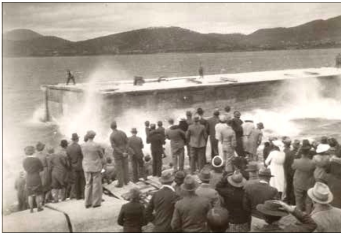
Launching a pontoon.
