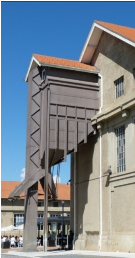
The ash bin, conveyor & chutes. Photo Keith Baker
