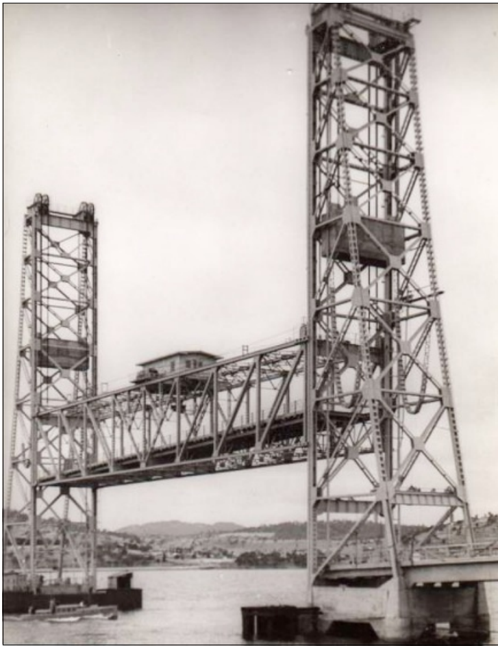
The floating bridge lift span opens for a tiny boat (bottom left) going downstream.. Note the operator's hut & the road deck sloping down from the land side (west) to the pontoon (east). Date & source unknown.
