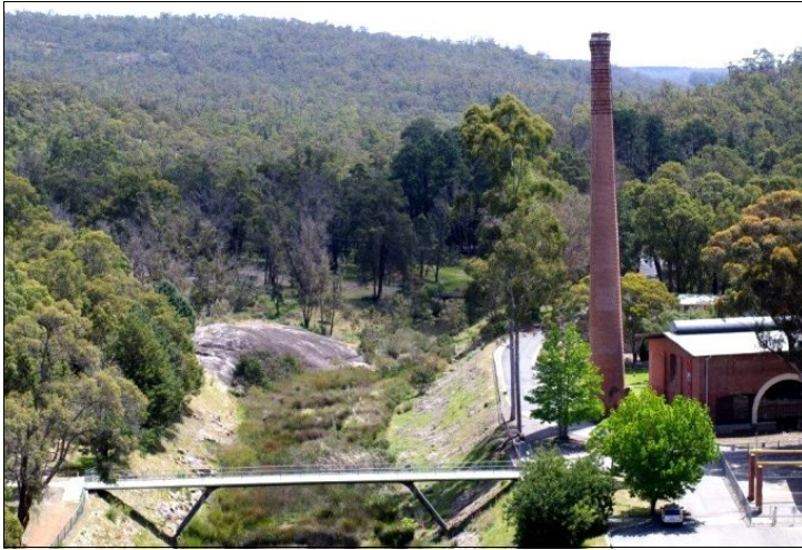
Helena Valley & the Goldfields Water Supply No.1 Pumping Station at Mundaring Weir. Photo: from Don Young.
