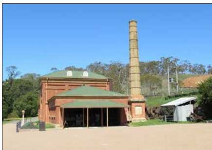
The Pumphouse at the Goulburn Waterworks supplied water to the town from 1886 to 1977.
