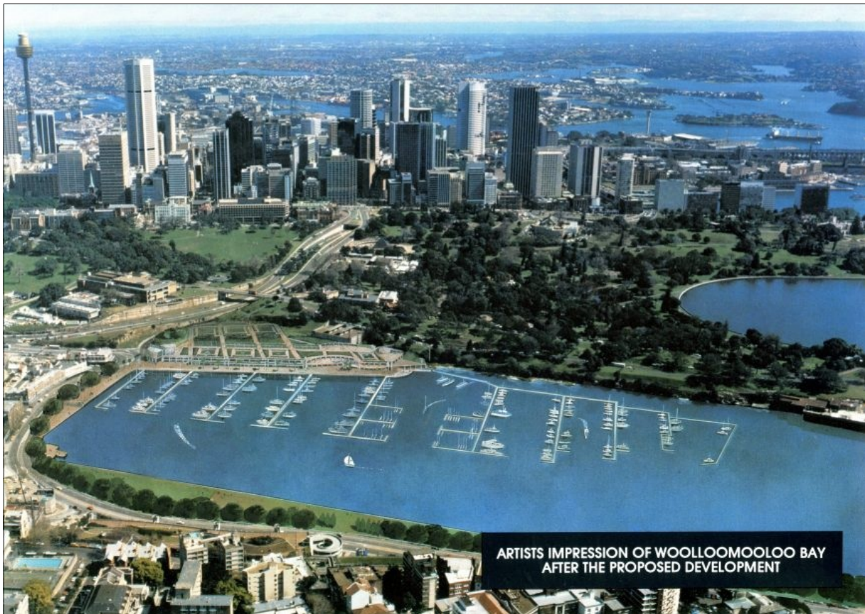
This "Artist's Impression" appears after the frontispiece (see previous page) of the EIS. It is slightly misleading, in that the number of boats shown in the marina is 180 rather than the 440 planned in the EIS, the marina doesn't project as far east as the footprint of the Wharf, and the busy Navy wharves have been turned into a peaceful, tree-lined park. Woolloomooloo Bay Developments EIS, Oct 1987.
