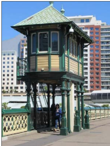
Operator's cabin for the Pyrmont Swing Bridge, which opened to let ships through to the end of Darling Harbour.
