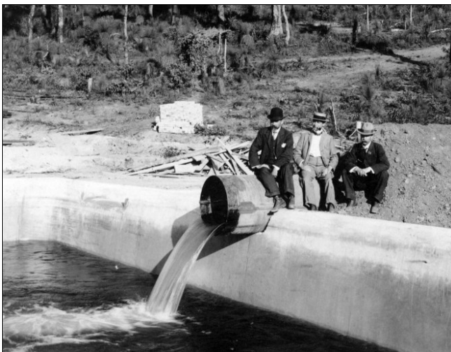
T. Hodgson, W. Reynoldson & E. Fenton at No.2 Pumping Station, 13 th April 1902, from Don Young.
