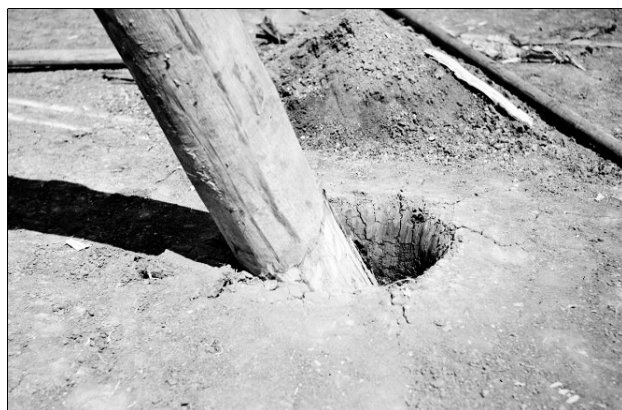
Stick Shed pole placed in its hole prior to backfilling, 1941 Photo: Culture Victoria
