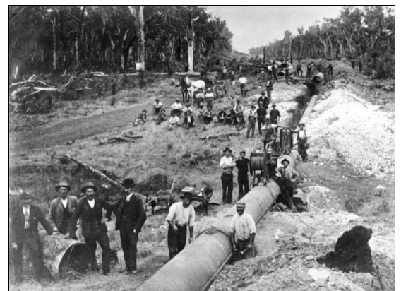
Laying pipe for the Goldfields Water Supply across the Darling Ranges. Photo courtesy the Forrest Family.
