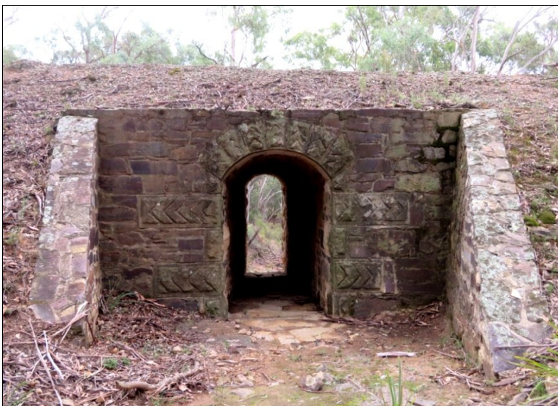
Another culvert near the Towrang Bridge.
