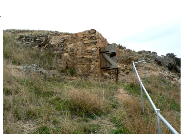
A relic of the Towrang Stockade – the Powder magazine under the bank of the Wollondilly River. Photo: N. Secomb for NSW OEH.
