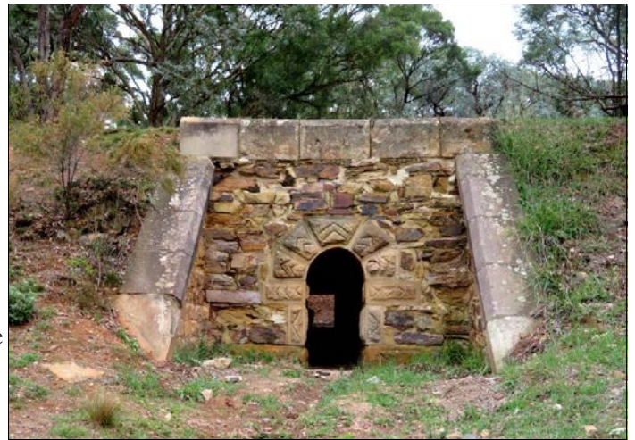
One of the surviving culverts near the Towrang Bridge. Photo: Frank Johnson.
