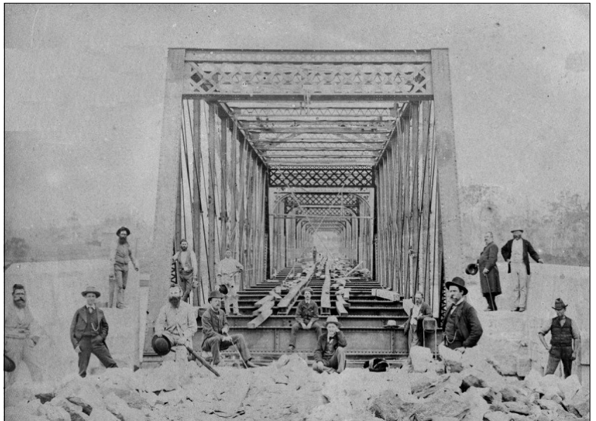
The timber floor of the bridge being placed. Photo source: Shoalhaven Historical Society.
