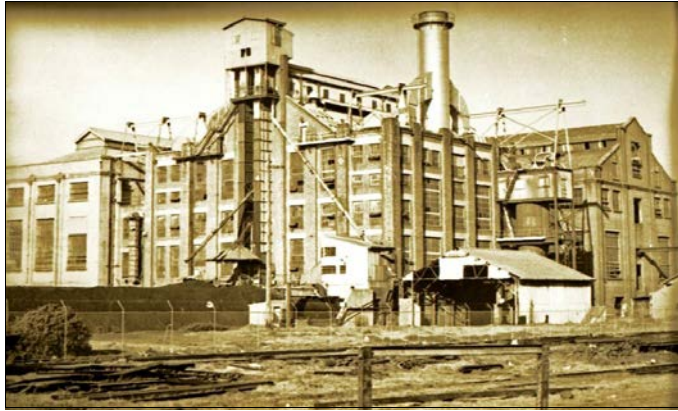
An undated photograph of the Zaara Street Power Station in Newcastle, photo by Bert Lovett. Source: Norm Barney collection, UofN Library.
