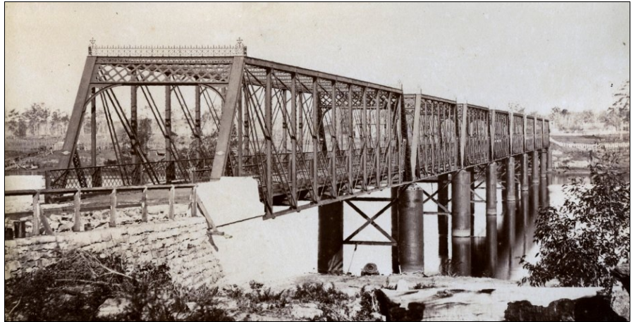
The Nowra bridge just before completion. The road surface on the northern approach is still being formed and the timber 'guard rail' is being painted. Note the different finished heights of the two nearer cast iron cylinder piers. Photo courtesy Shoalhaven Historical Society.
